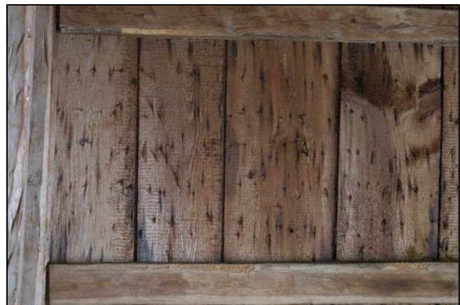
Figure 32: Detail of roof sheathing with hand-hewn rafter at left, roof purlins at top and bottom of frame, and water-power sawn sheathing boards at middle
