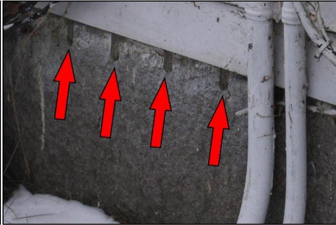
Figure 10: Plug and feather marks in granite underpinning
