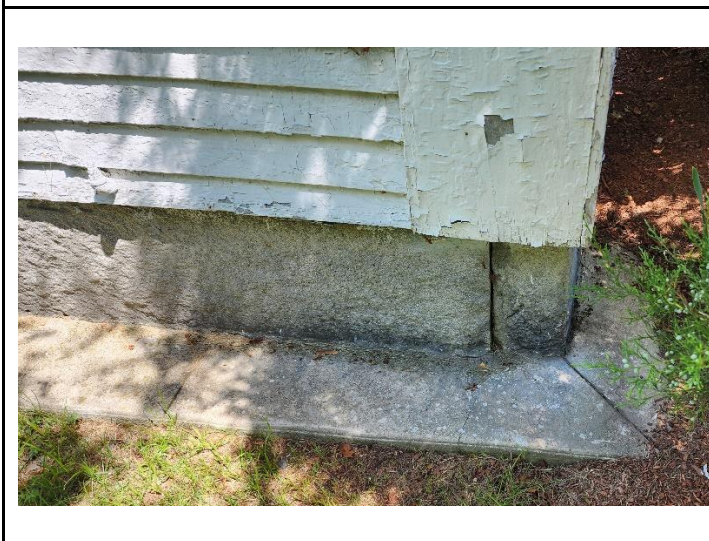
Photo 24: Granite block foundation with concrete skirt
