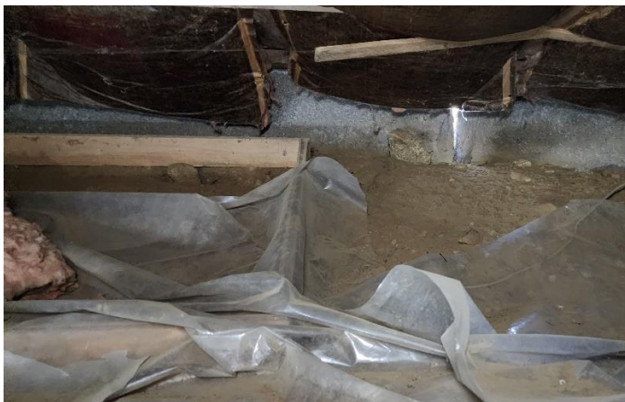
Photo 21: Openings between granite block foundation
