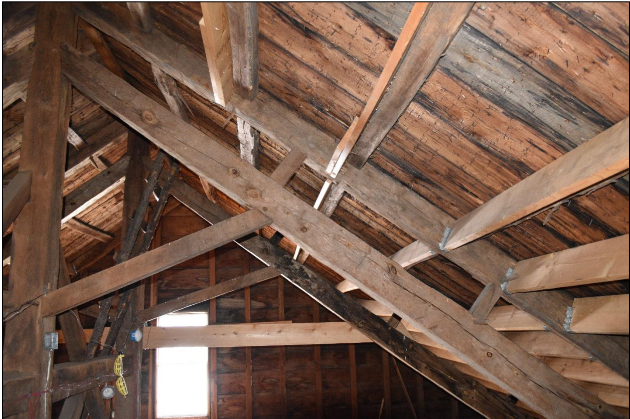
Figure 35: View of attic, facing east, showing modern framing that has been added to the historic frame
