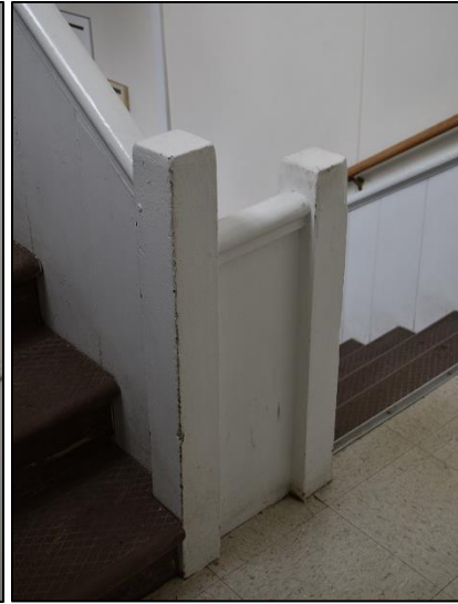
Figure 22: Detail of landing newels
