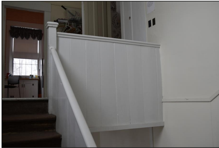
Second floor landing and solid half wall with integrated handrail, looking easterly (Photo by M. Williams)
