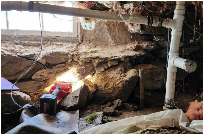
Photo 20: Stacked stone foundation under granite block
