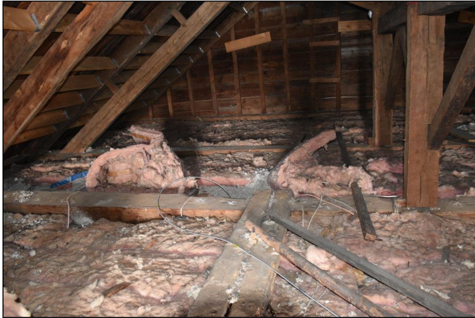
Old, disturbed attic insulation, looking west (Photo by M. Williams)
