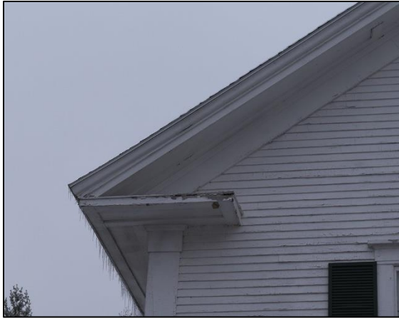
Figure 9: Detail of eave return
