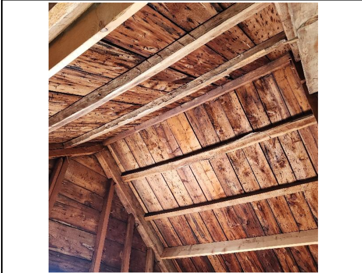
Photo 12: Upper section of the roof without the sistered 2x10's
