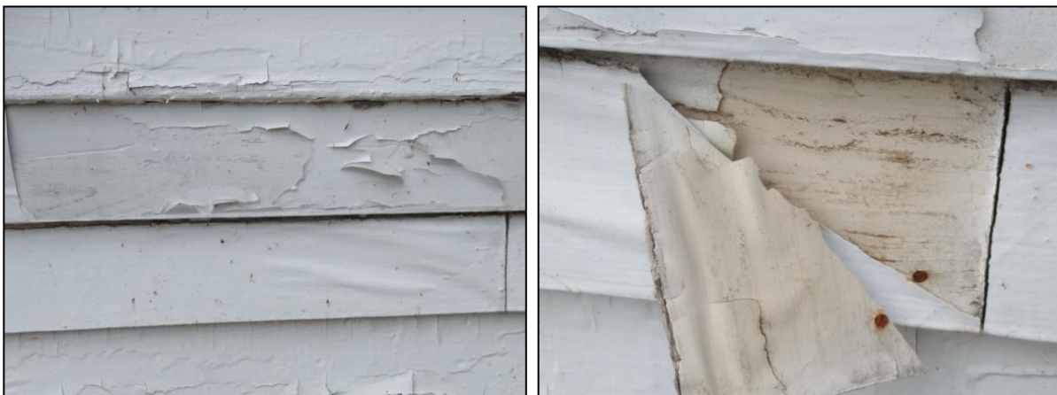
North side peeling paint on clapboards
