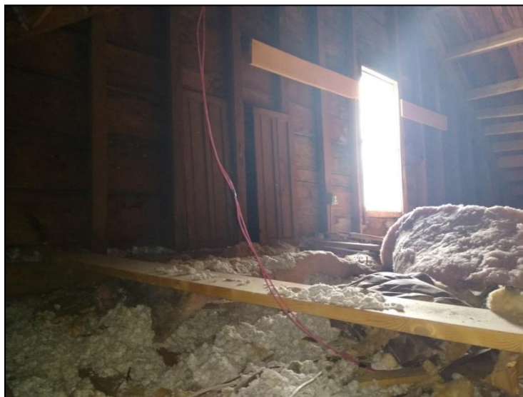
Old, disturbed attic insulation, looking east
