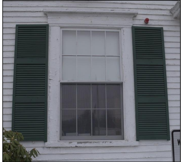
Figure 12: Typical Town Hall window
