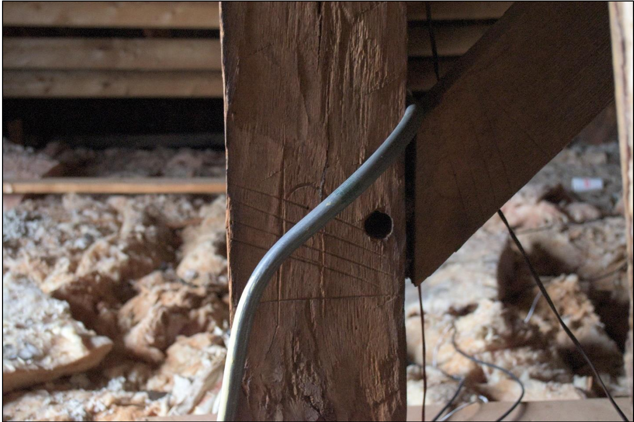
Figure 31: Numerals inscribed in the scribe-rule frame at either side of a joint allowed the master-builder to reassemble the individually-carved members of frame he created on the ground when the building was raised.
